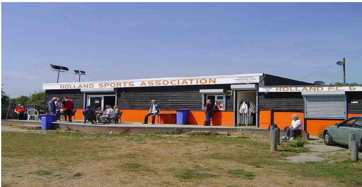
Dulwich Road pavilion
